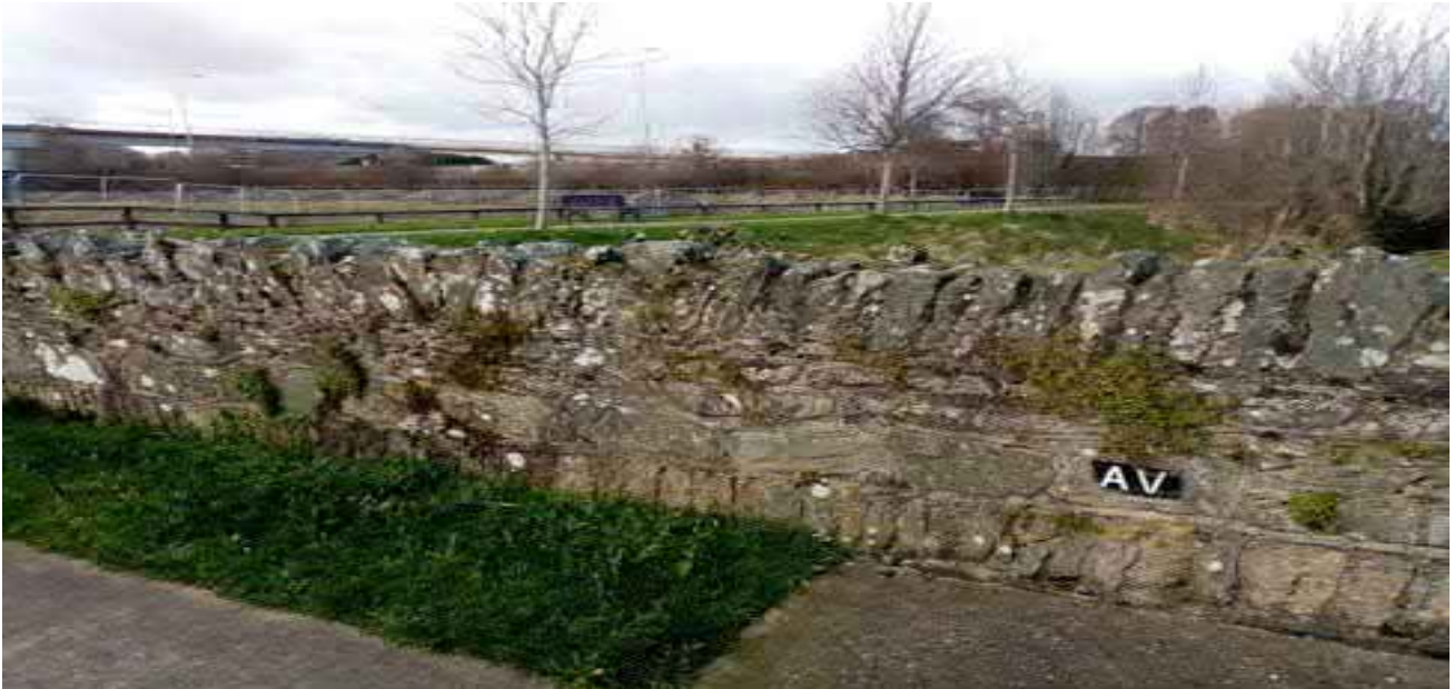
Figure 5: Bridge infrastructure in place at Johnstown
